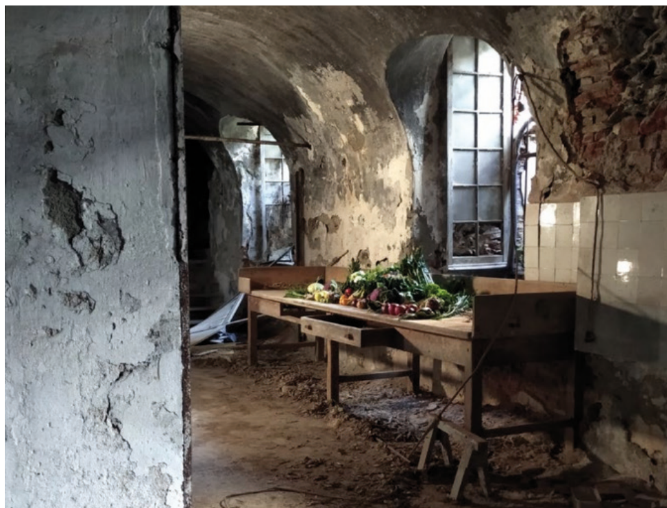
▲ Interior space: disused underground kitchens of the Albergo dei Poveri.
