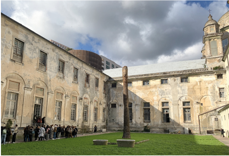
Views of the underused south-west courtyard flanking the church main nave. photo: E. Sommariva, 2024
